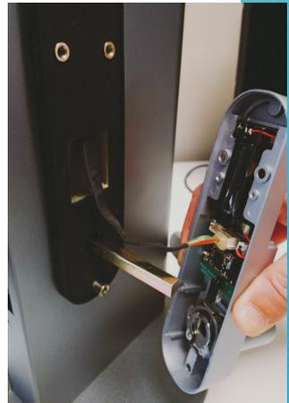
5 Attach the inner unit to the bracket by using the 3 shorter machine screws. The longer one goes below the spindle. The remaining two shorter ones go in the upper corners inside the battery compartment.
